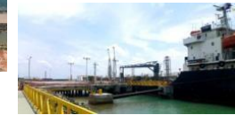
Berth 4 ( liquid jetty ) - for liquid cargo
