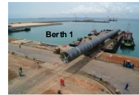
Berth 1 ( length 130 m ) - for Tug & barges up to 2,000 DWT with water draft up to 5m LWS
